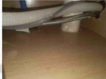
Water staining and damage observed under sink cabinetry.
