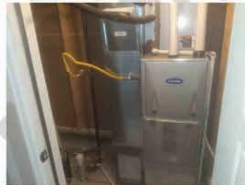
Water staining and damage observed on sill plate.
