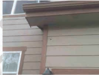
No rain gutters observed on top story of structure.
