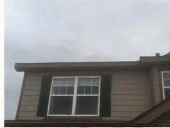
No rain gutters observed on top story of structure.
