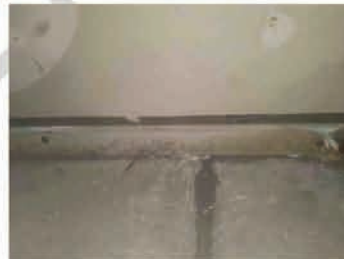
Mold-like growth observed on drywall common Utility Closet.
